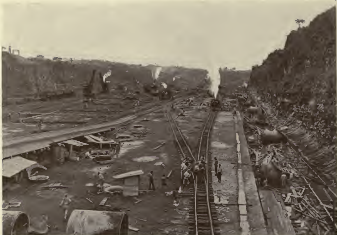
Installing concrete floor and lateral culverts. The circular holes in the floor are to admit the water to all the locks. The floor varies in thickness from 13 to 20 feet of solid concrete.
