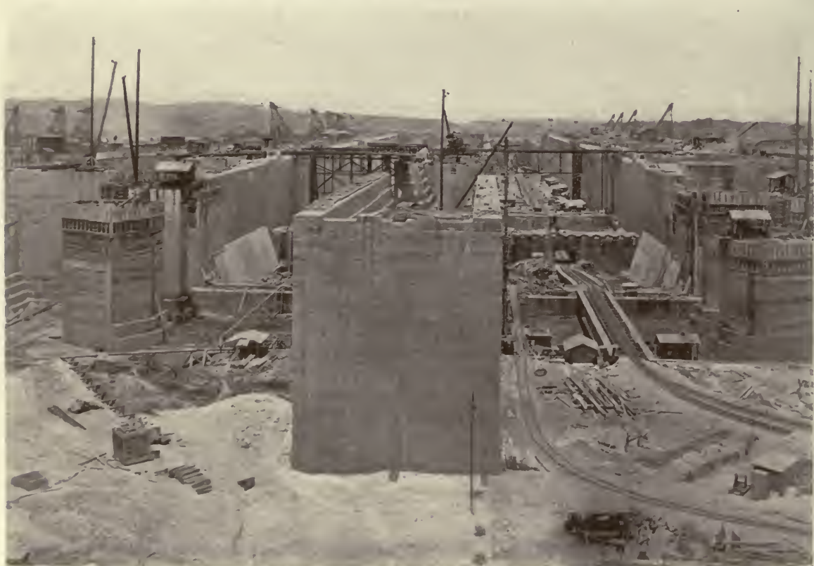
The locks are in pairs, so that if any lock is out of service navigation will not be interrupted. One also may be used for the ascent and the other for descent of vessels. The locks are 110 feet wide and have usable lengths of 1,000 feet.
